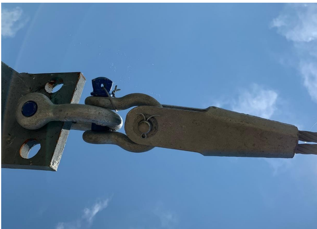
Figure 1: Rope connection with a rope lock and shackle
